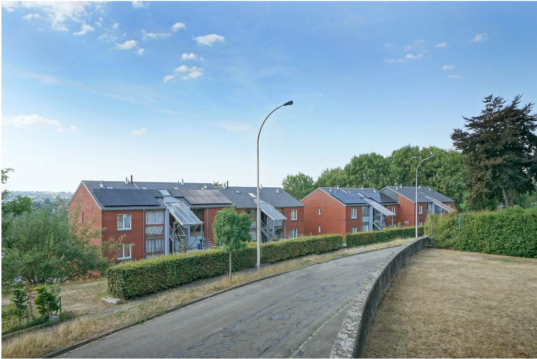
FIGURE 1 – Installation des panneaux photovoltaïques - rue.
