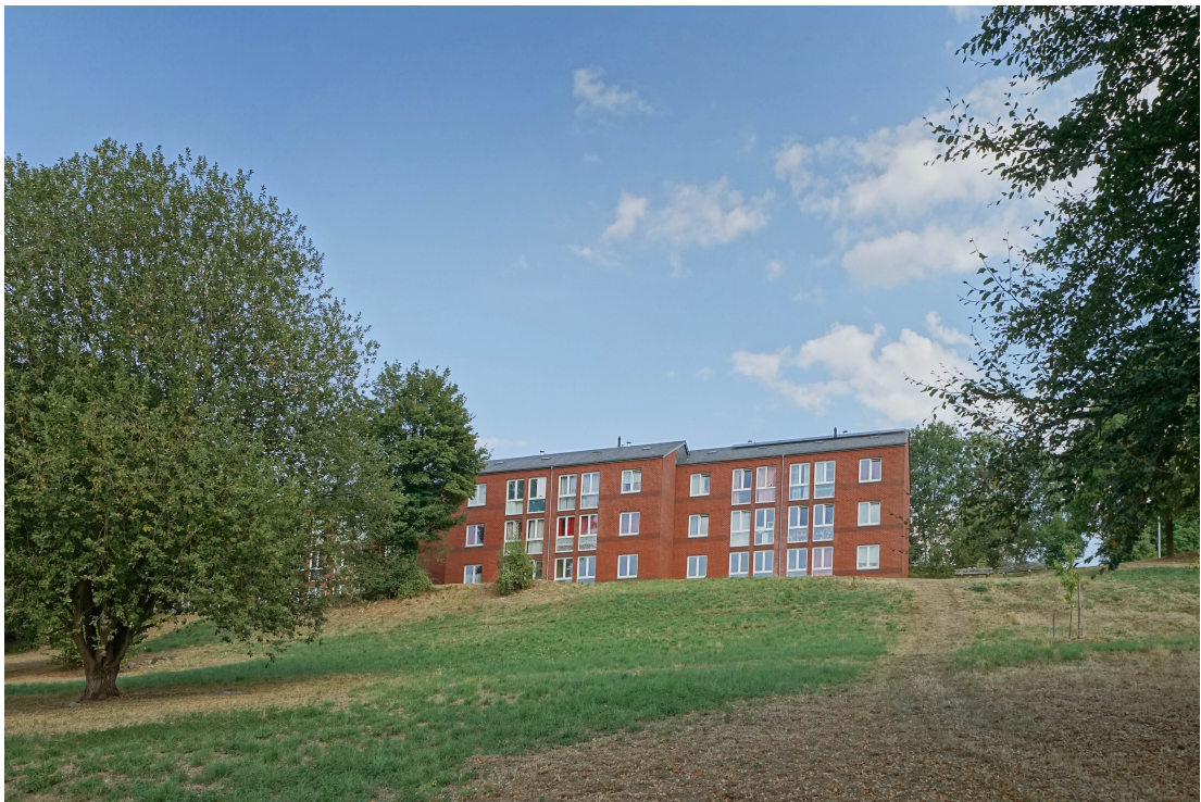
FIGURE 2 – Installation des panneaux photovoltaïques - jardin.
