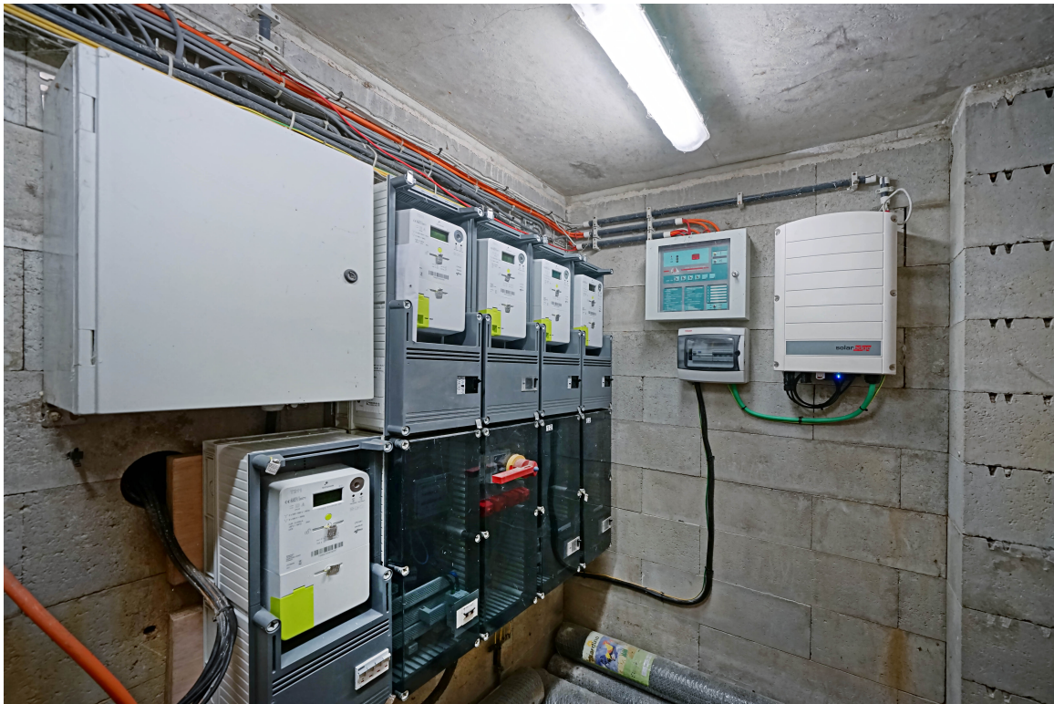
FIGURE 3 – Installation des panneaux photovoltaïques - local commun.
